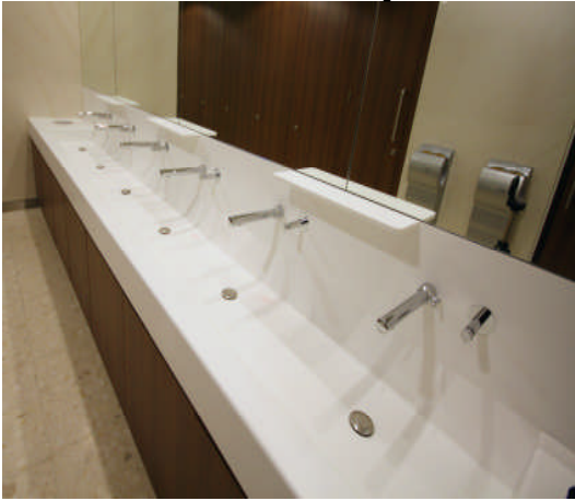
Bank Canary Wharf - Levada trough- Corian
