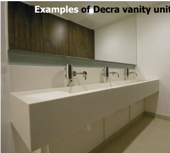
Levada trough vanity unit Abbeygate House
