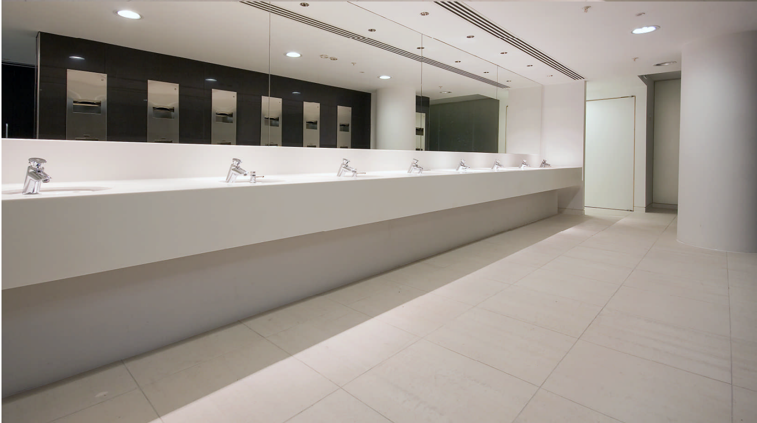
Selfridges staff washroom vanity units in Corian Cameo White. Installed by Decra Ltd. Architect; Gensler; M/C Ibex Interiors March 2008.
