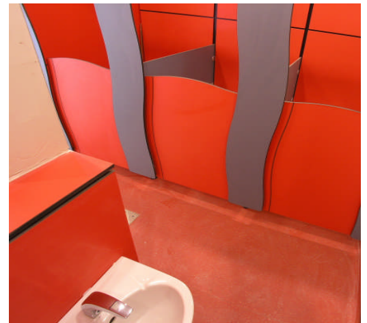
Project completed August 05
