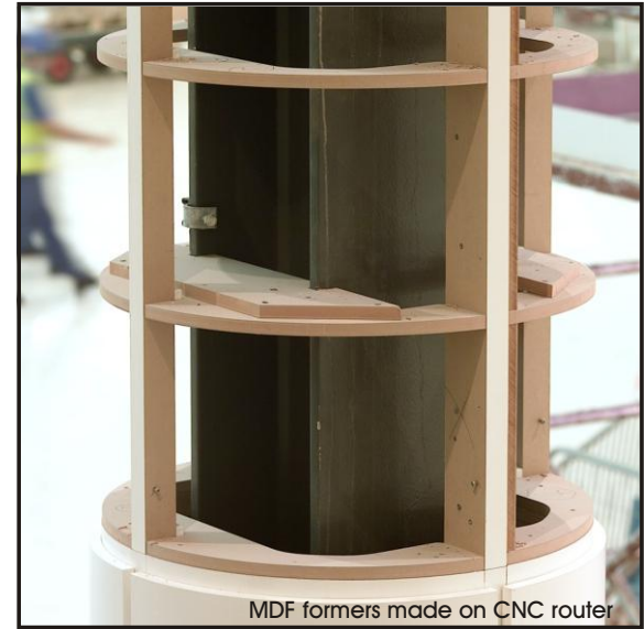
Gatwick Airport North Terminal Column cladding
