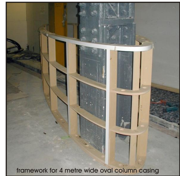
Gatwick Airport North Terminal Column cladding
