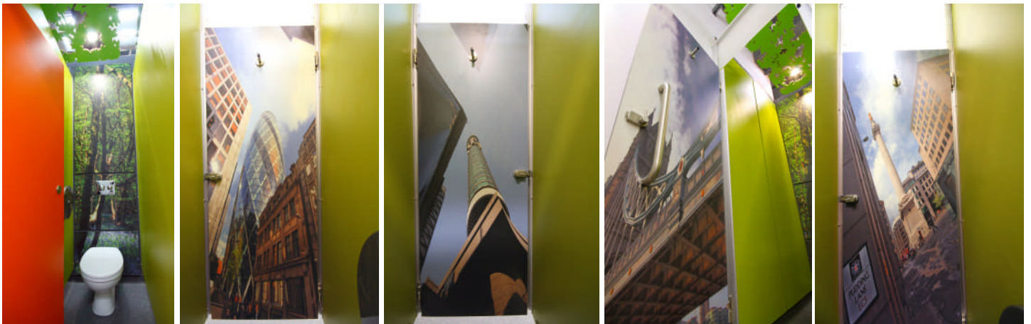
Rear duct panels and door reverse panels are faced with woodland theme images for the ducts and iconic London images for doors - melamine protected as Formica laminates
