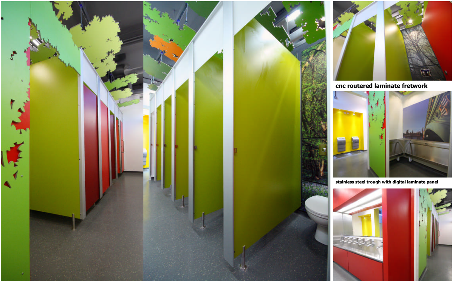
Earlham primary school Forest Gate aluminium pilasters, multi colour doors with Perspex over panels
