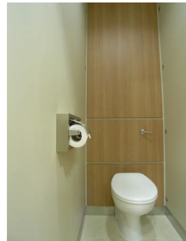
Partition panel installed into channel sections and clad with s/steel
