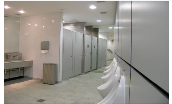
Stratum 20mm cubicles and 13mm solid grade laminate urinal duct panels
