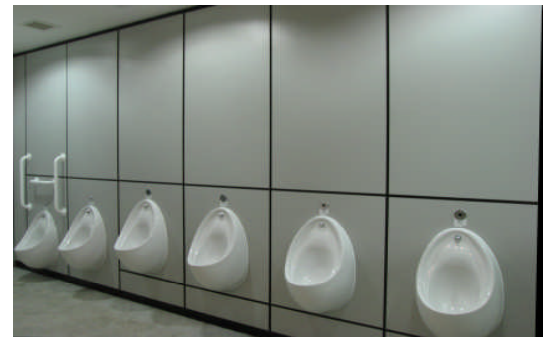
Urinal duct panels
