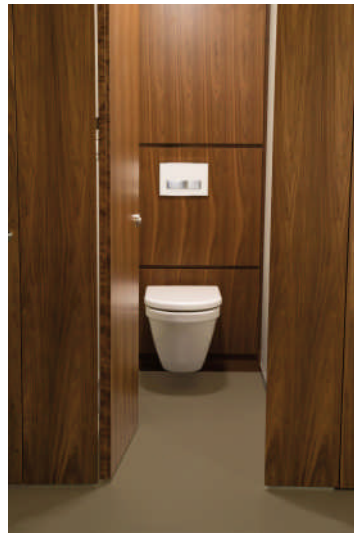
Burj in black walnut fascia and duct panels
